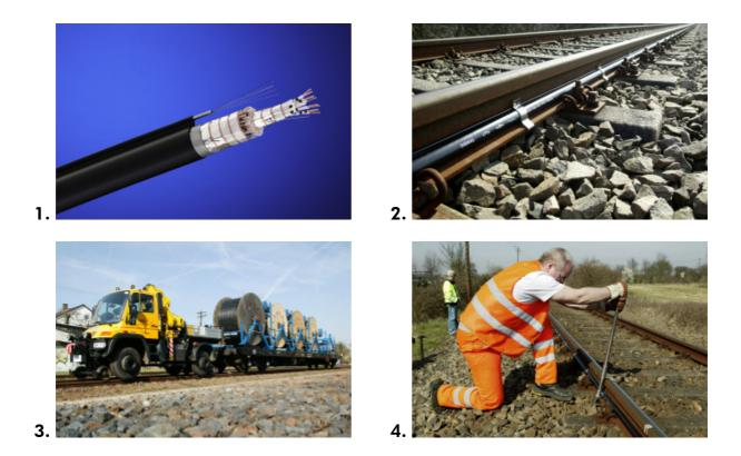
DuoTrack<sup>®</sup> is an innovative all-in-one system solution for quick, cost-effective and long-term railway cabling for non-electrified regional railway lines. Top left: the DuoTrack<sup>®</sup> cable; bottom left: laying the cable using the special vehicle; bottom right: attaching the cable with special holding clamps produced by Contec; top right: the laid cable.
