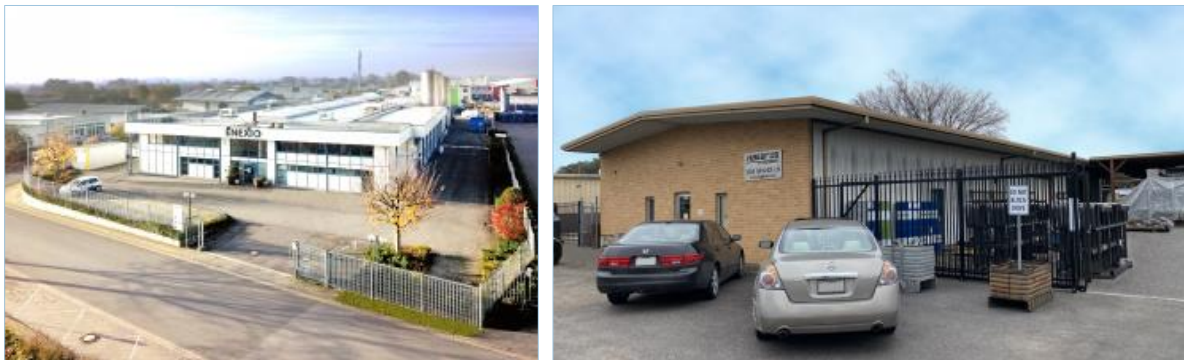
Buildings of ENEXIO Water Technologies (left) and Hagbros Precision (right) (Pictures sources: ENEXIO Water Technologies / Hagbros)
